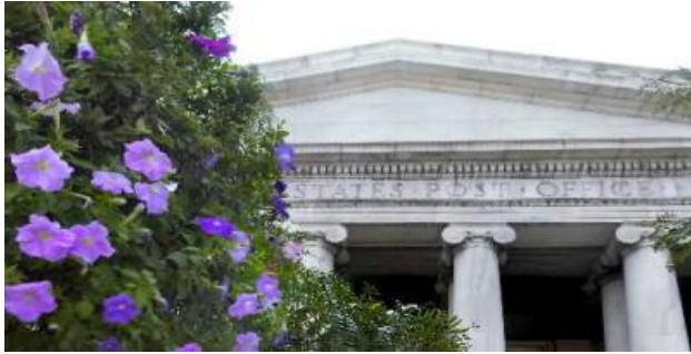
York's downtown post office on South George Street was commissioned by Congress in 1912 as a memorial to the Continental Congress being held in York. Post office officials recently announced that the building was for sale, raising concerns among the city's architecture preservationists. (Daily Record/Sunday News -- File)
