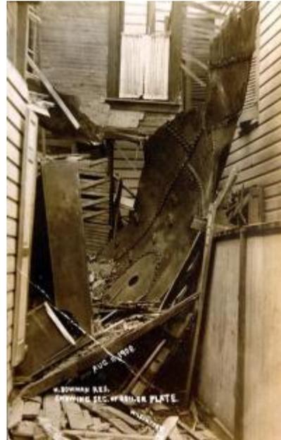
This is a piece of the boiler that flew through the air and crashed into a home on North Queen Street. The piece went through the roof and hit a dresser in a bedroom, according to 'The Gazette' at the time.
